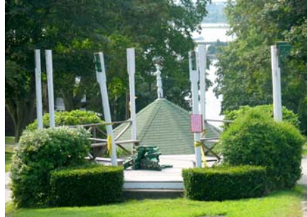
The Gazebo "in progress"
